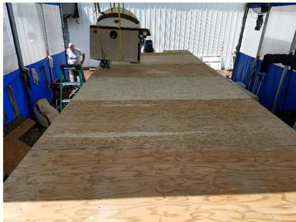
Deck removal and new plywood flooring
